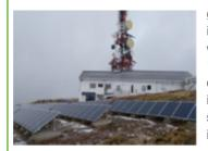
Cellnex is implementing a solar energy self-generation project in Spain, which involves the installation of solar panels at 692 rural sites with which it expects to produce around 3GWh/year of 100% emission-free energy at the point of consumption, reducing distribution losses. The solar initiative in Spain is launched with the aim of using self-generation of energy as a lever to capture inefficiencies and reduce the carbon footprint.
